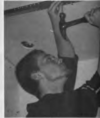
Senior Sean Dieter hammers nails into the drywall.
